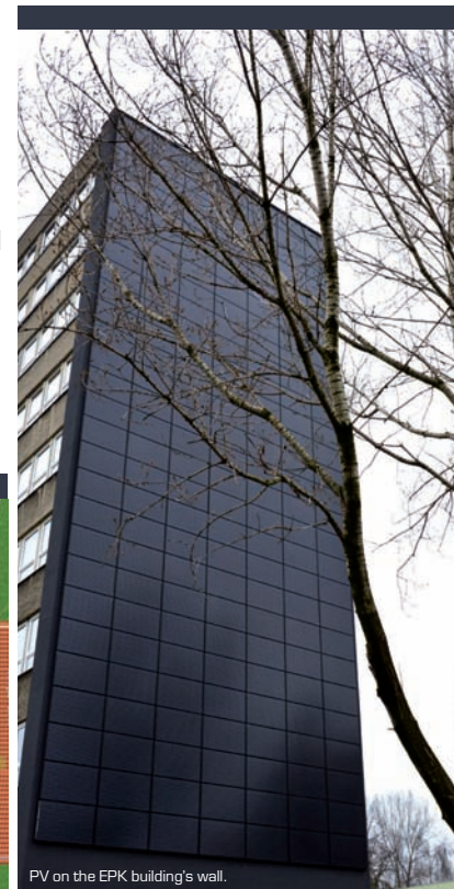
PV on the EPK building's wall.
