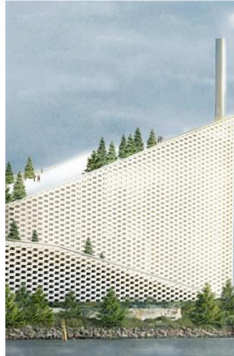
Waste incineration plants
